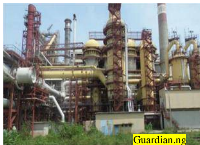
Plate 9. Ajaokuta Steel Company (Blast Furnace section)
