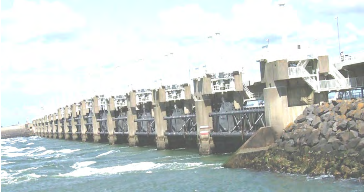
Plate 1: The Formidable Haringvliet Dam at the mouth of Rhine River, South-west Netherlands. (Note that the North Sea lies to the left side of this imposing structure; Shot was taken by the Author during a study trip in 2008).
