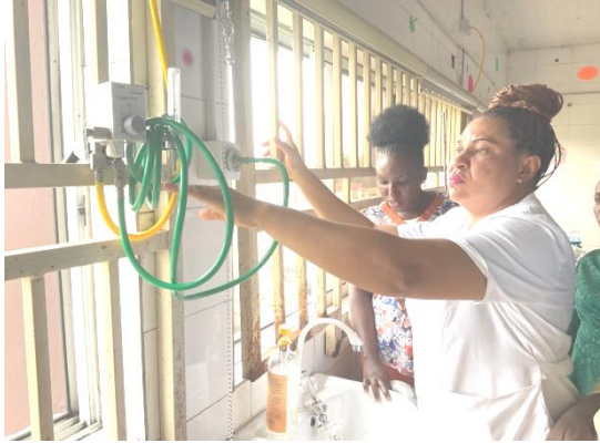
Fig 18: Blended air -oxygen terminal in SCBU
