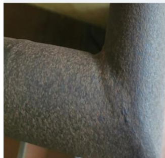
Corroded railing
