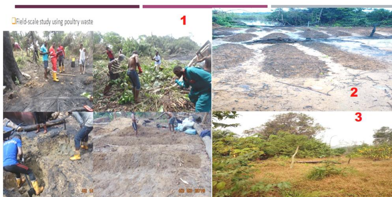
Plates 1&2. Site mapping, clearing, excavation and ridge making during field-scale bioremediation of Ngia Ama polluted land, Rivers State, Niger Delta in 2018 with my PhD students and community youths; Plate 3 full biodiversity restoration 307 day post-remediation
