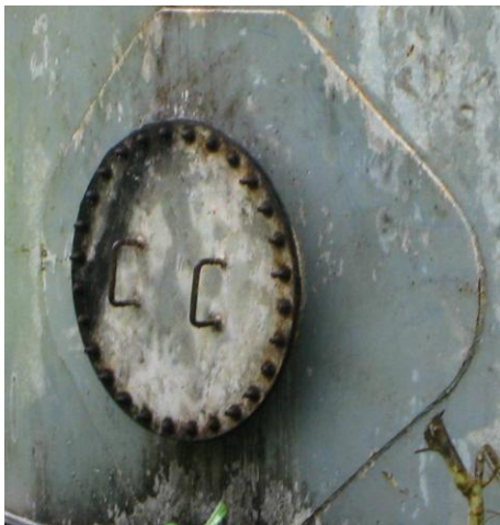
Figure 10c Man hole for maintenance work
